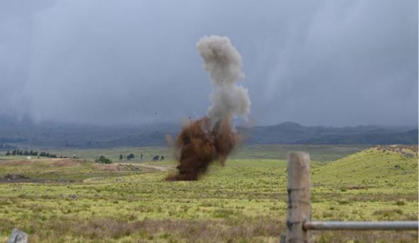
Disposal of high explosive munition via controlled detonation
